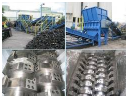
Fig. 9. Installation for rubber pyrolysis
