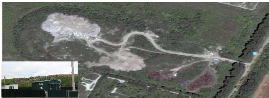
Figure 1. Municipal solid waste landfill and operating biogas combustion plant (Kamianets-Podolsky, Ukraine, 2022)
